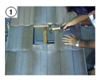
**2A.** Straight bonded roof:-Knock tile lugs off bottom of tile in the course above to allow the tile to sit flush with the vent.
