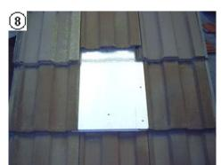
**9.** Pull the tile/s back into position, smooth the silicon out to close all gaps between vent and tile/s (*Be careful not to block out any water courses*). Finally, run a bead of silicon down both sides of the vent attaching the tiles to the vent. The water courses above vent may also be silicon sealed if preferred.
