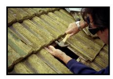
**3.** Knock a lug off each tile in the course above to allow both tiles to sit flush with the vent. (You will have a spare roof tile to every vent you place)
