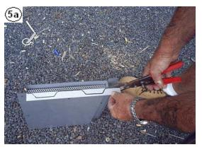
**5.** Trim vent along texta mark with tin snips, when this is trimmed it will fit the profile of your roof and will also leave a flap of metal to the right hand side of the vent which when fixed in the roof will fit under the tile at the right hand side of the vent. Be sure not too cut too much material away.
