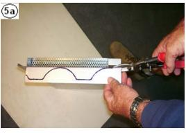
5. Trim vent along texta mark with tin snips, when this is trimmed it will fit the profile of your roof and will also leave a flap of metal to the right hand side of the vent which when fixed in the roof will fit under the tile at the right hand side of the vent. Be sure not too cut too much material away.
